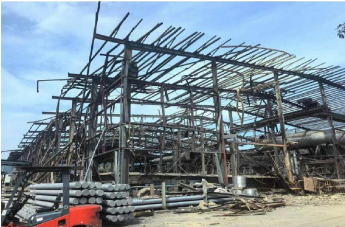
Figure 5. July 9, 2024 Fujian Province explosion.
